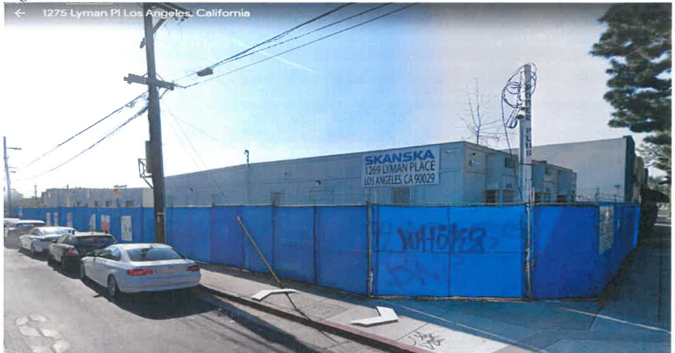
Photo above: Illegal modular office buildings operated by Hollywood Presbyterian.
